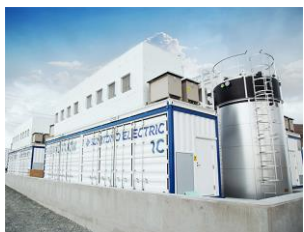
Storage battery for grid stability
